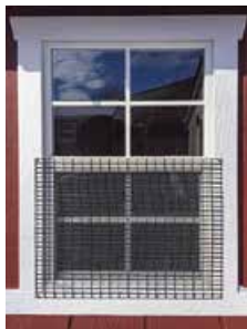
Wire Over Windows
