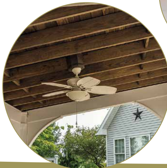
VINYL SANTA FE Underside of Roof
