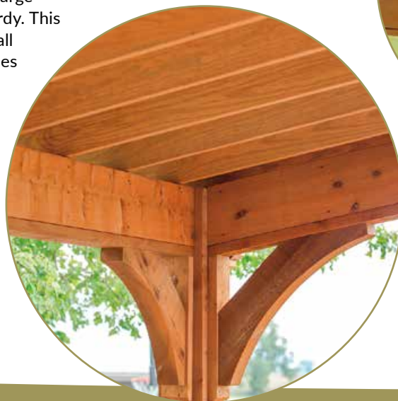
CEDAR SANTA FE Braces & Underside of Roof
